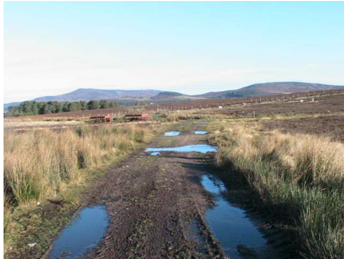
Fig.3 - Photo taken looking north. Shows poor drainage on the track
